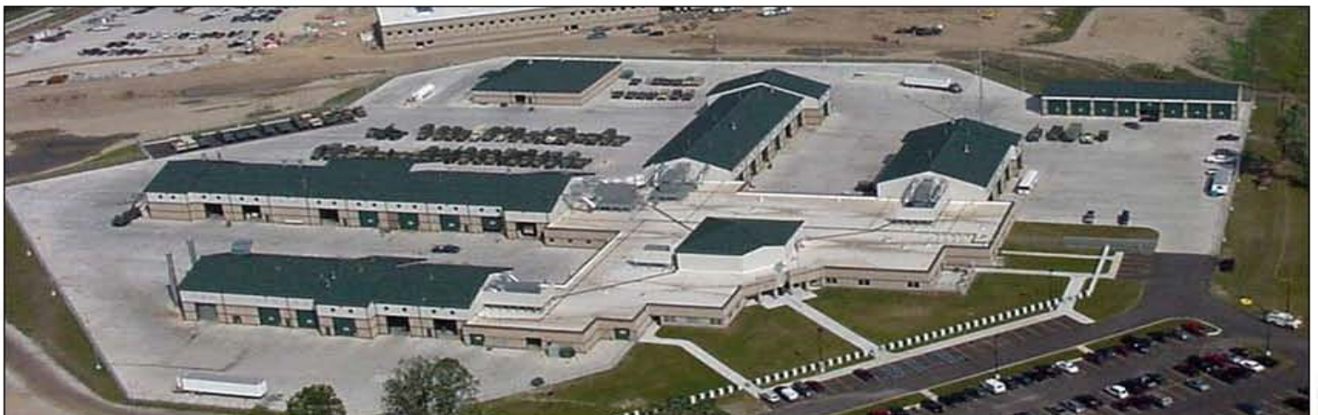
An aerial view of the CSMS located at the Michigan National Guard's Headquarters Complex in Lansing, Mich. The MIARNG CSMS paints and processes 12 to 15 vehicles/pieces of equipment every month and provides the only full re-painting services for the MIARNG. In addition, the Allied Trades Shop manages sheet metal repairs and weapons storage/shipping containers for mobilization and annual training.
